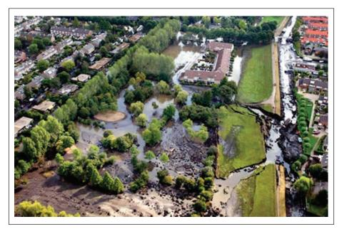
**Figure 1.** A Levee Failure in Wilnis, the Netherlands Note:This levee breach was caused by the drought in the summer of 2003.
